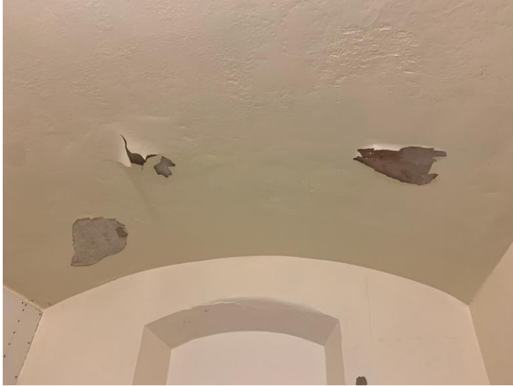
PEELING PLASTER AND PAINT IN CELL
